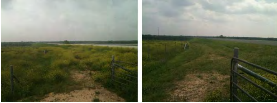
Dam Maintenance at Dam 1 – Before and After
